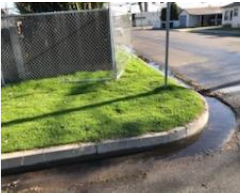
Location of Thirteenth Street and Kings Avenue where an ADA curb ramp would need to be installed along with sidewalk.
