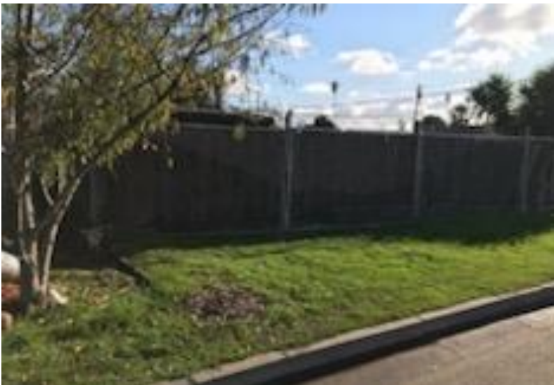
A view of the side of the property along Thirteenth Street where sidewalk would need to be installed.
