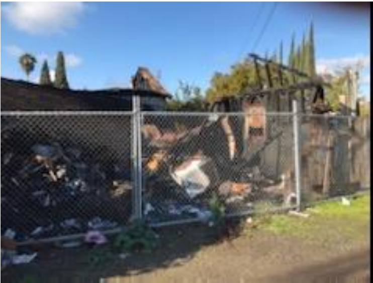
Debris from the fire that would be required to be removed as part of the rebuild.
